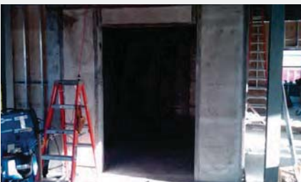
BABB Security crew installing a new modular vault.
